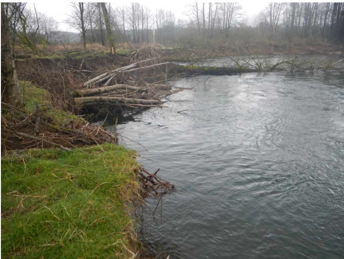
Figure 10: Riprap failure at upstream end of Port of Grays Harbor Well site revetment (photo date: February 13, 2013).
