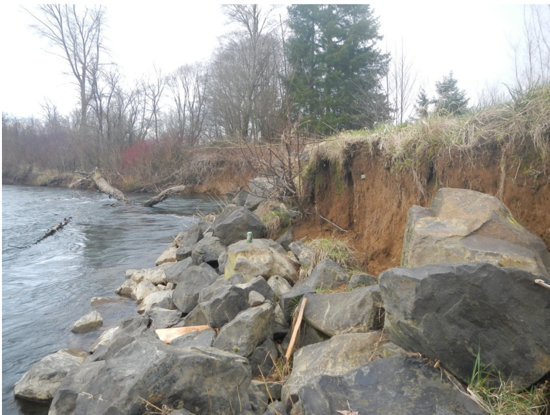
Figure 10: Riprap failure at upstream end of Port of Grays Harbor Well site revetment (photo date: February 13, 2013).
