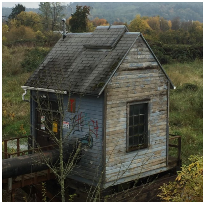
Old Pump – 1940s
