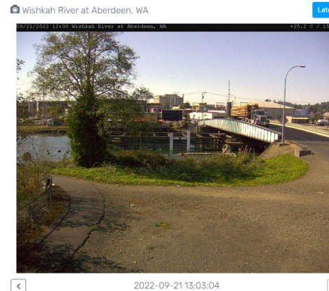
Looking at downstream face of Heron St. bridge
