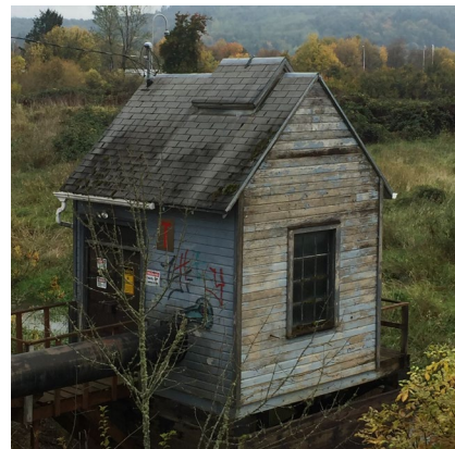
Old Pump – 1940s
