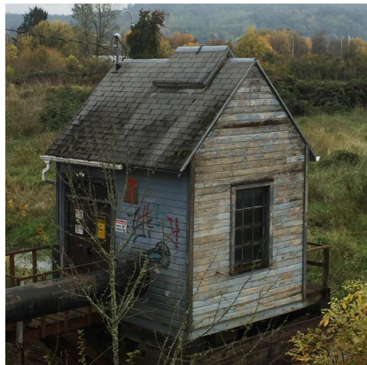
Old Pump – 1940s
