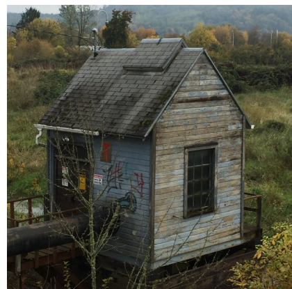
Old Pump – 1940s
