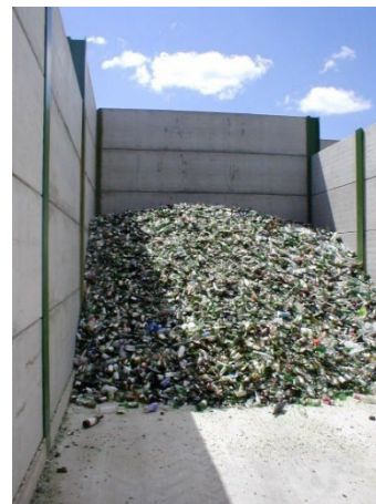
Figure 8: Glass Storage Bunker
