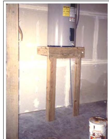
Elevating the water heater and furnace are easy and inexpensive examples of wet floodproofing.
