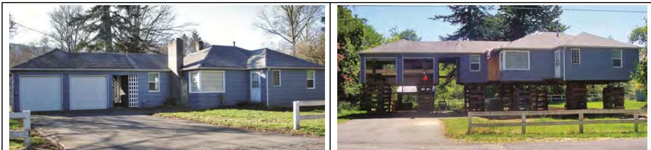
The standard elevation technique is to jack the structure above the flood level and then construct a supporting wall.
