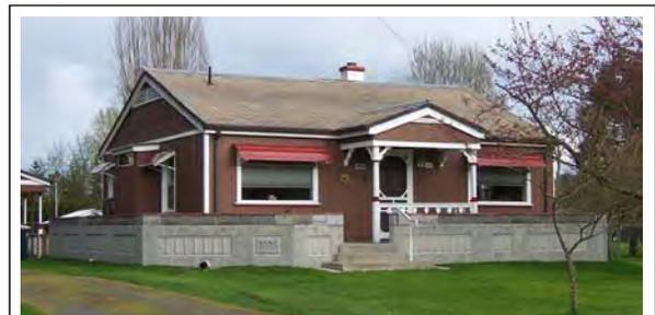
The owner of this house in Centralia built this floodwall around the house after his first flood. It has worked during subsequent floods.
