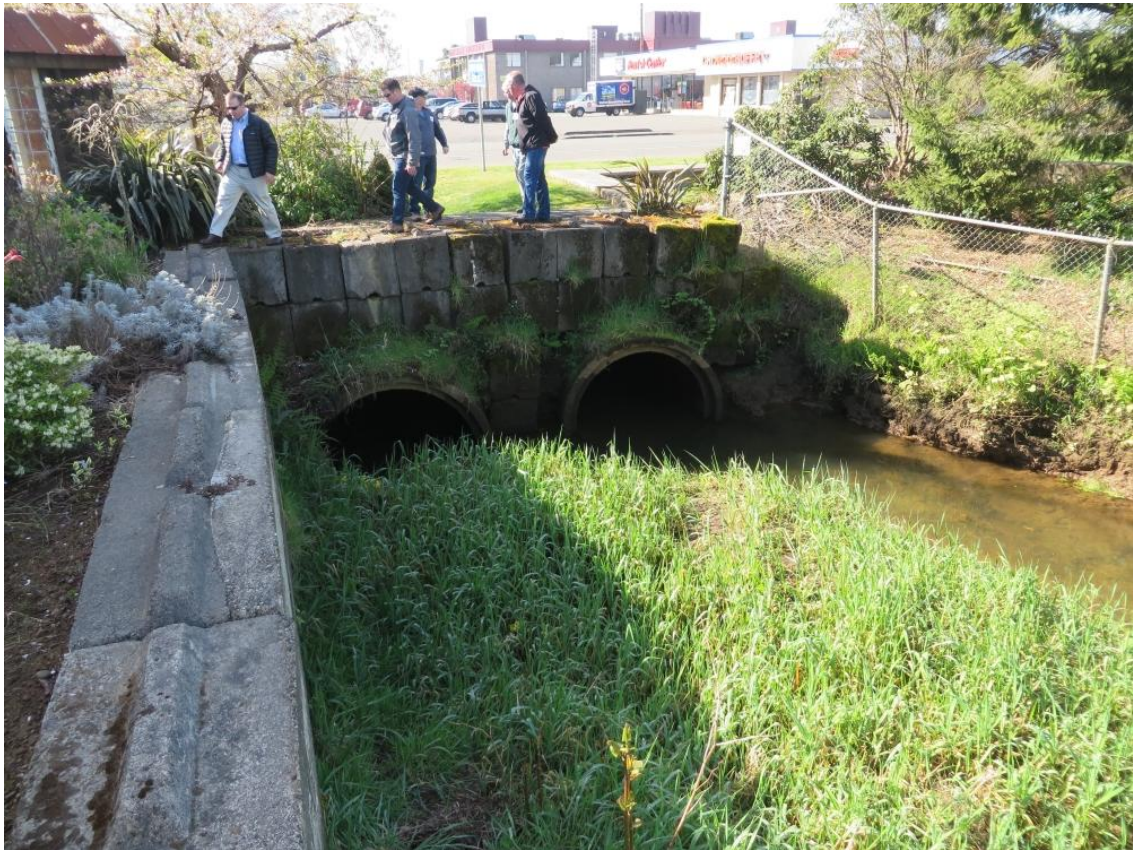
FRY CREEK - CULVERT CONSTRICTIONS
