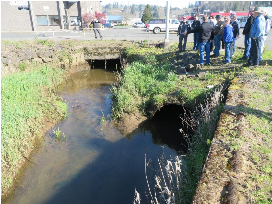
FRY CREEK - CULVERT CONSTRICTIONS
