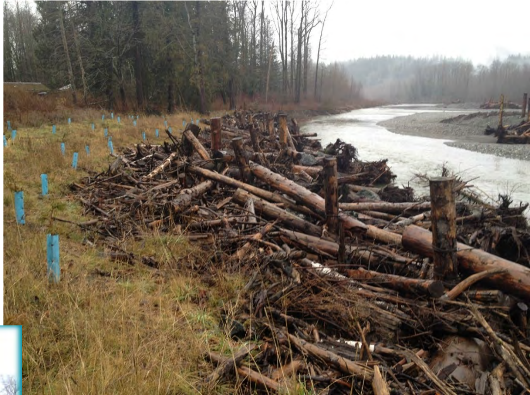
Complex timber revetment on South Fork Nooksack. View is downstream. Photo taken ~2012 by T. Abbe
