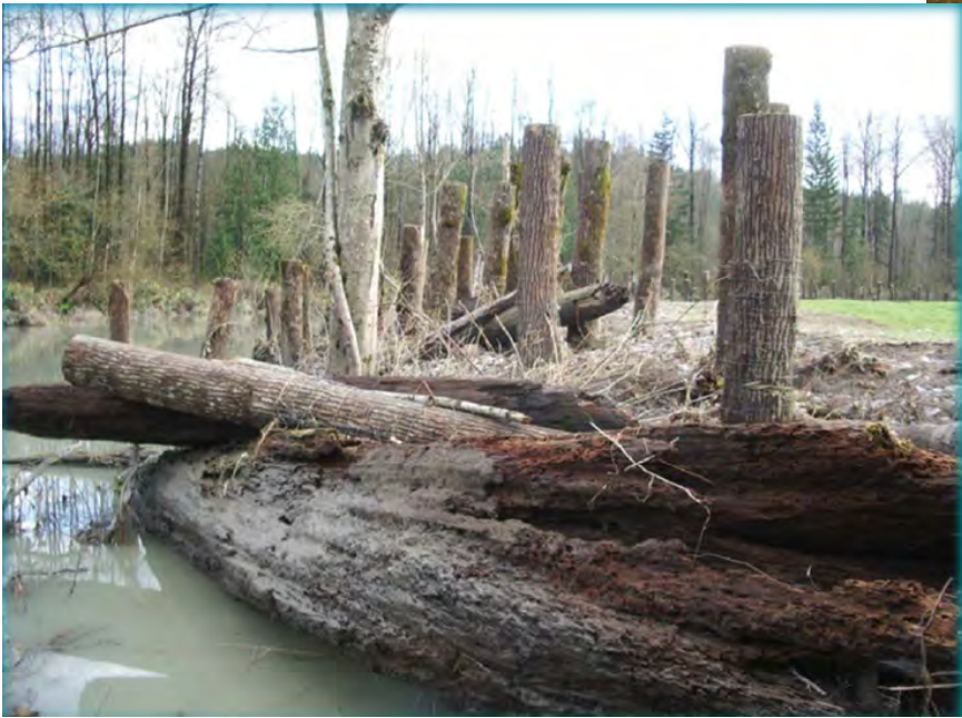
(8) Flood fence revetment taken by Aldrich and DeVries 2017
