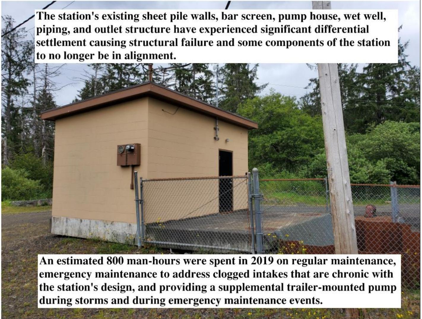
**An estimated 800 man-hours were spent in 2019 on regular maintenance, emergency maintenance to address clogged intakes that are chronic with the station's design, and providing a supplemental trailer-mounted pump during storms and during emergency maintenance events.**
