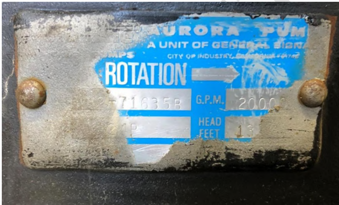
Figure 3-2. Existing 100 hp Pump 1 tag
