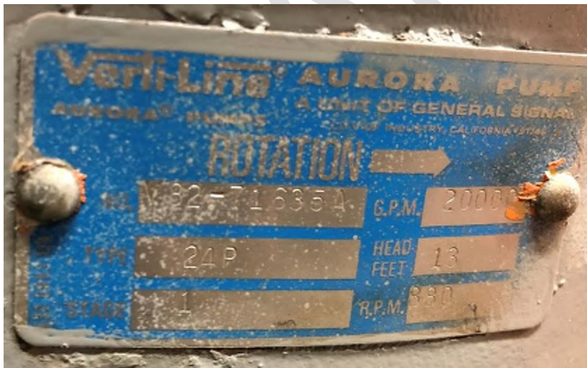
Figure 3-4. 100 hp Pump 2 tag
