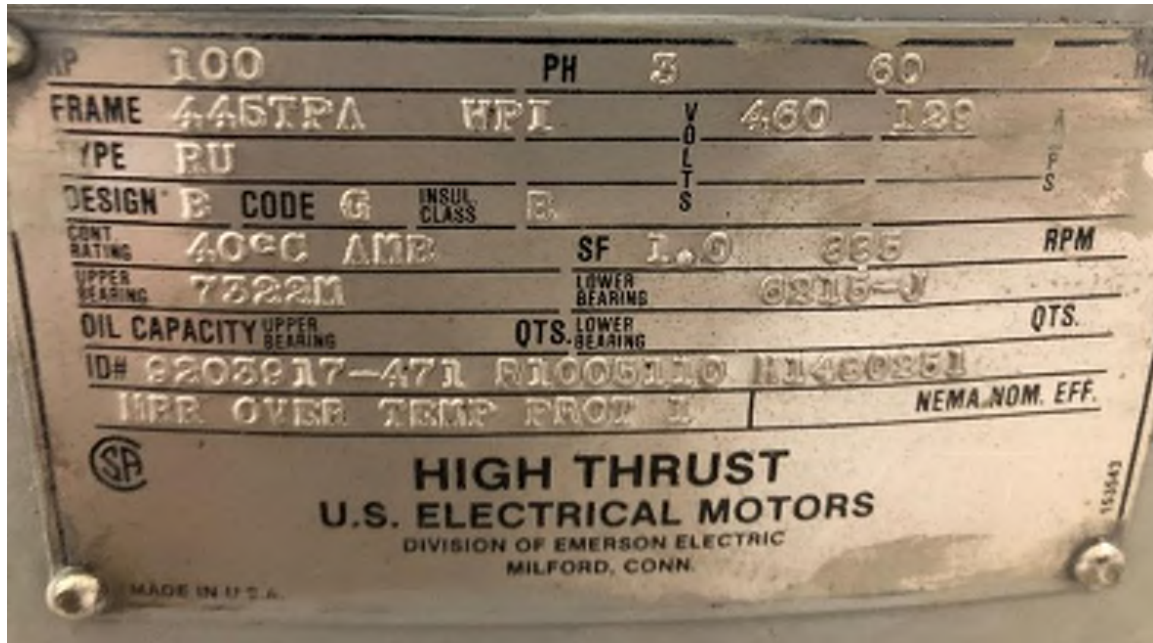
Figure 3-5. 100 hp Pump 2 motor tag
