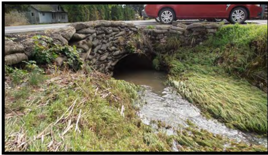
Upstream view of CMP arch culvert, Ribelin Road near Cascade Hardwood's office
