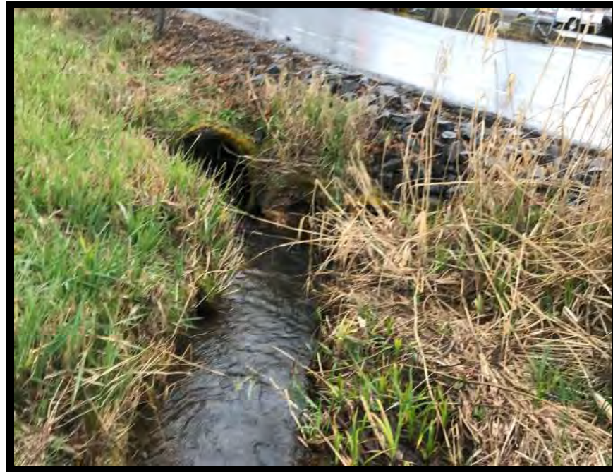
Upstream view of twin 24-inch concrete culverts, Ribelin Road
