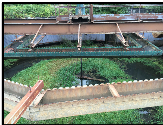
ACTIVATED SLUDGE TANK
