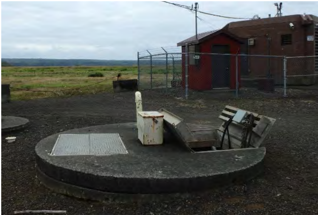
Figure 2-1. Existing K Street Stormwater Pump Station
