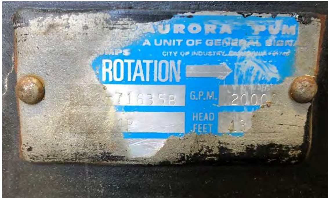
Figure 3-2. Existing 100 hp Pump 1 tag
