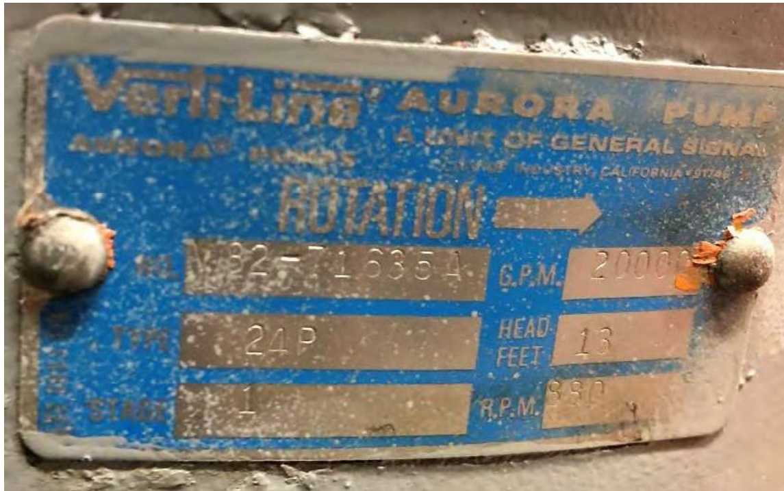
Figure 3-4. 100 hp Pump 2 tag
