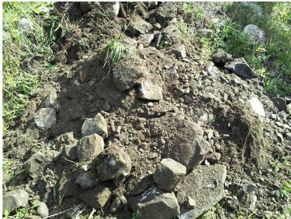
Figure 19. Example of basalt quarry spalls material in the southern dike surface.
