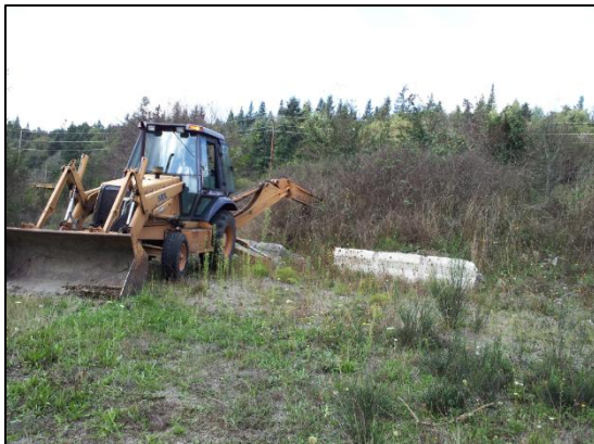
Figure 15. Excavating for sampling in the northwestern stockpile; An example of native soil materials above..
