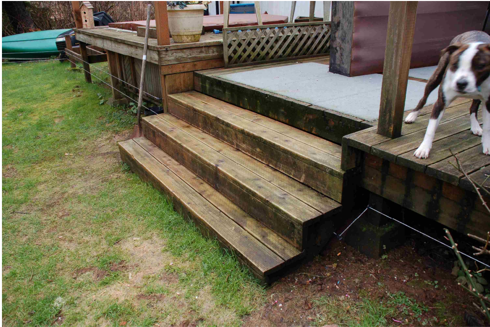
Front deck steps. According to the owner, during periods of flooding the water has come as high as the third step (from the bottom).
