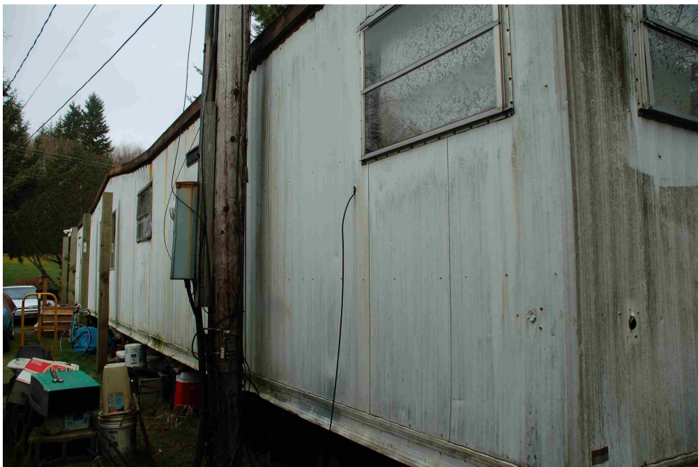
Rear of the manufactured home. The skirting was all washed away in a flood event in the last ten years (or so).
