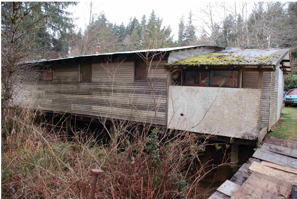
Rear of large wood-frame storage building. According to the owner, in the same flood season that swept away the skirting to the trailer the foundation of this structure was undermined and damaged. As shown, there is a small creek or slough that is under the riverside edge of the structure.
