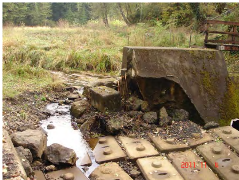
Photo 4: Mill Creek Park Dam temporary repairs after breach, facing upstream (HDR 2013).
