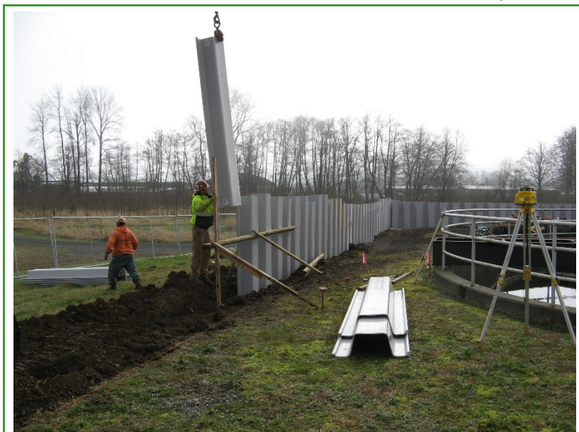
Figure 4. Sheet Pile Wall Construction at the Montesano Municipal Wastewater Treatment Facility in 2014.
