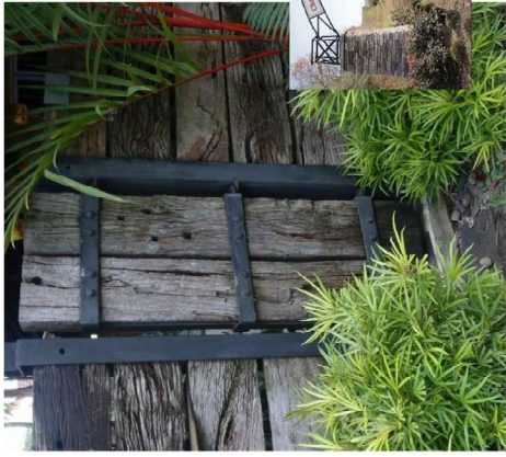
FENCE WITH RAIL ROAD SLEEPER FENCE POST
