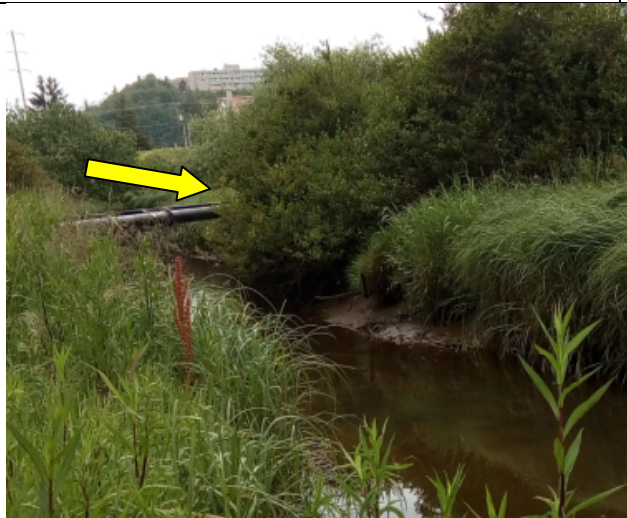
Image 3. View of Fry Creek looking upstream from proposed levee crossing. Arrow indicates general area of inflow channel to storage pond. The bottom of the utility pipe seen in the image is about 8.5 ft elevation. All managed and natural (below the 100-year flood event) water levels will occur below this pipe.
