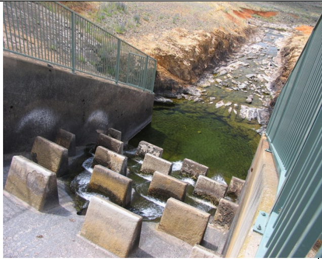
Image 9. A concrete baffle drop is positioned at the pump's drainage culvert and serves to dissipate the energy as pumped water is introduced to the estuary.
