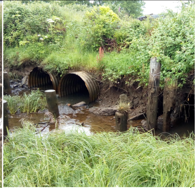
Image 2. The proposed site of the tide gate structure and box culvert. This view is looking downstream at the culverts located under the railroad tracks. The two (2) culvert rounds and one (1) concrete box culvert (right of image next to piling) will be replaced by the culvert/tide gate system.
