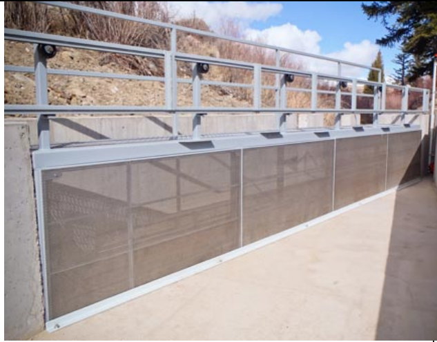
Image 5. Panel fish screens similar to what would be in place at the diversion channel. Design would include catwalk for maintenance and angle to 20 degrees to help with debris and leaf litter removal. Proposed length is about ½ of what is pictured here.
