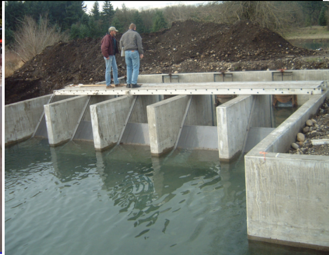
Image 6. Inclined screens allow easier cleaning from atop and push floating debris up and over screening adding a self-cleaning element. In this example the screen mesh size is very small. For Fry Creek the screens at the storage pond inlet channel will be removable horizontal panels with width designed to divert the 100- yr flood event.
