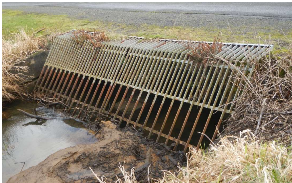
Figure 5 – The entrance to the Cherry Street culverts is protected by a trash rack.
