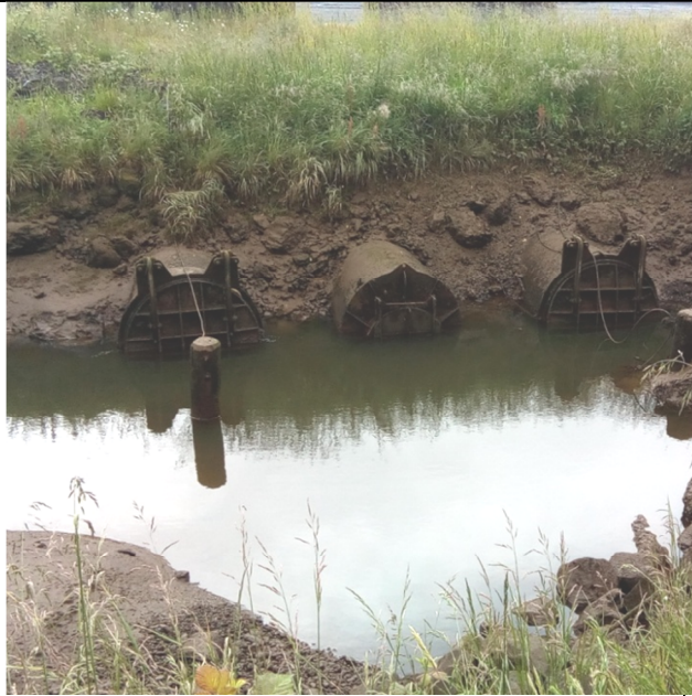
Image 1. Existing Fry Creek tide control structures include three (3) 6-ft diameter culverts whereby the far left culvert serves as the creek outflow during ebb tide after the other gates close. A flap-gate in the middle culvert and cables on the others allow adjustment to increase ebb tide (outgoing) conveyance.
