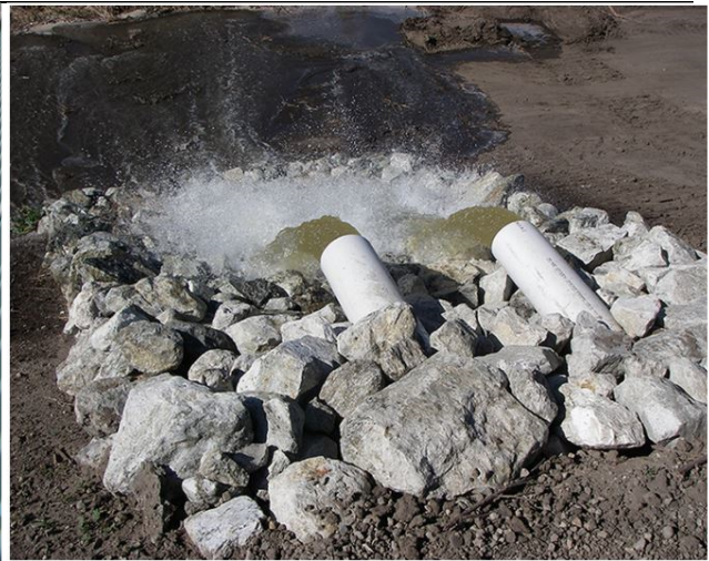
Image 10. Rip rap may also be used to line the outlet channel as a somewhat more natural way to dissipate energy.
