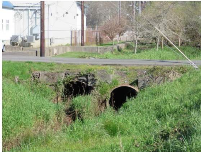
FRY CREEK - CULVERT CONSTRICTIONS
