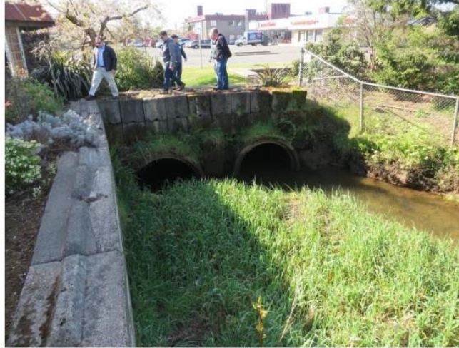
FRY CREEK - CULVERT CONSTRICTIONS
