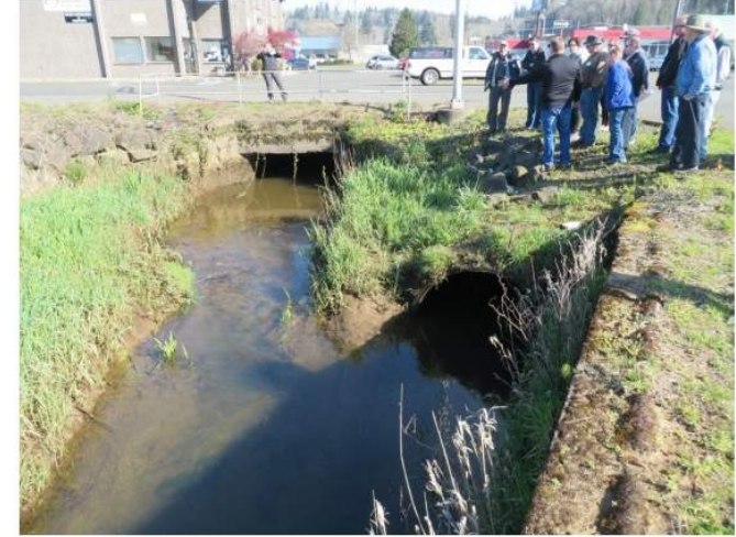
FRY CREEK - CULVERT CONSTRICTIONS
