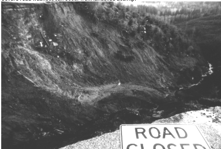
Severe road washout can occur from landslide activity.
