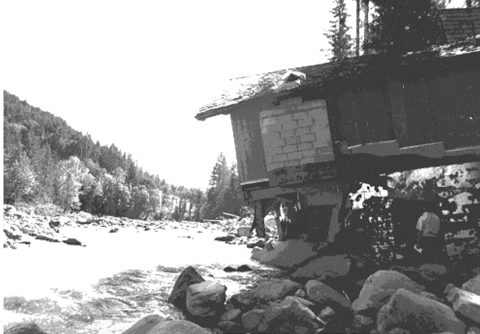
One of six homes destroyed by eroding floodwaters in Canyon Creek, Whatcom County.
