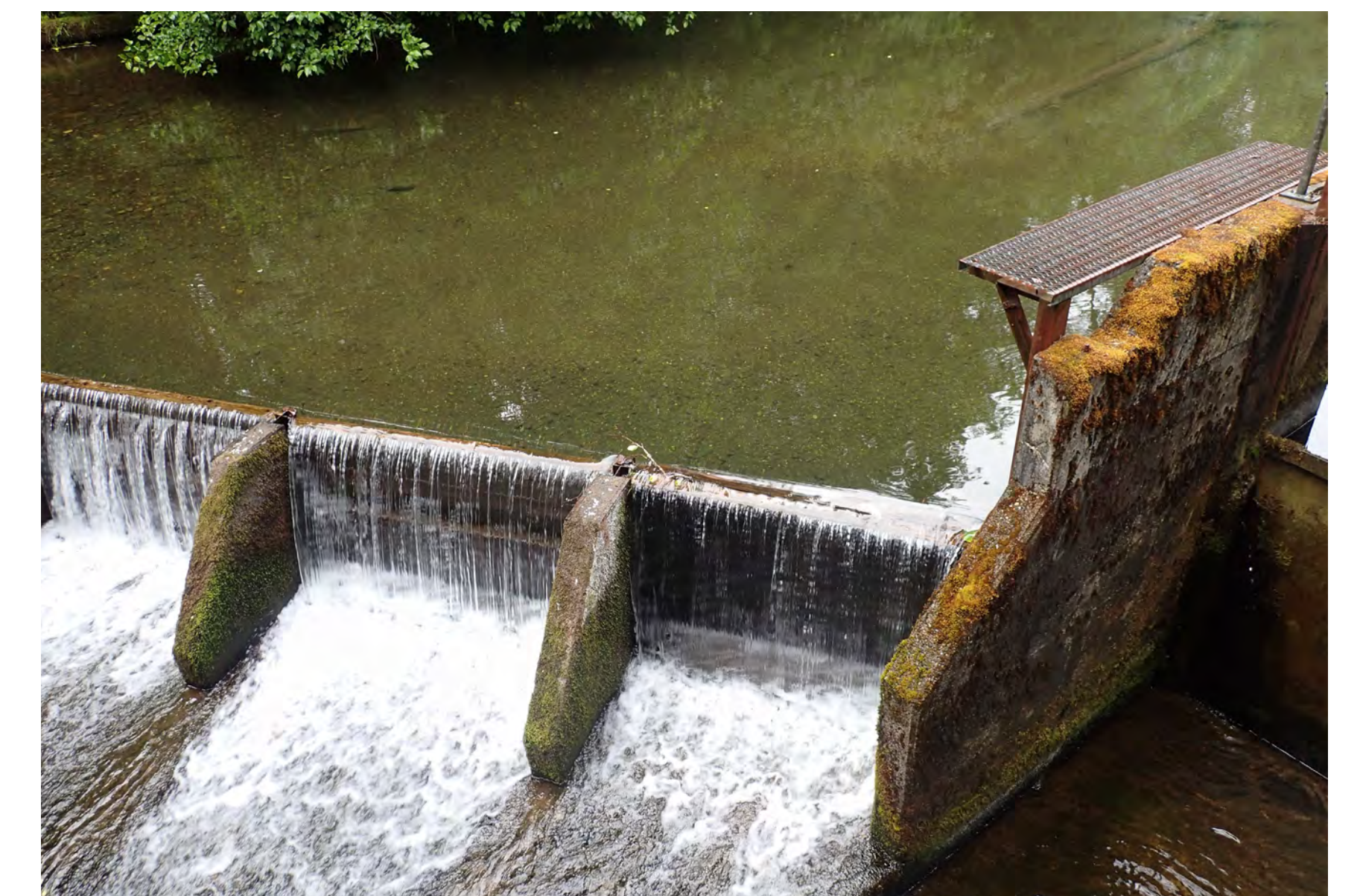
This fish barrier on Bingham Creek is impassable has a fish ladder and smolt trap that has provided approximately 40 years of wild coho life cycle monitoring information.
