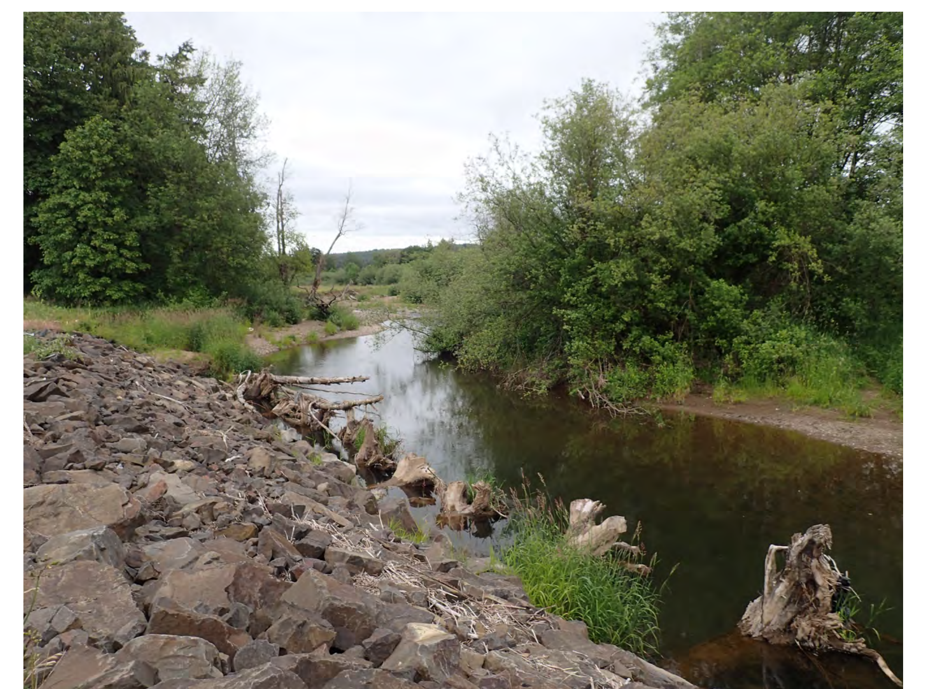
Infrastructure in the floodplain has disrupted natural processes, as illustrated by this riprap embankment protecting a bridge crossing.
