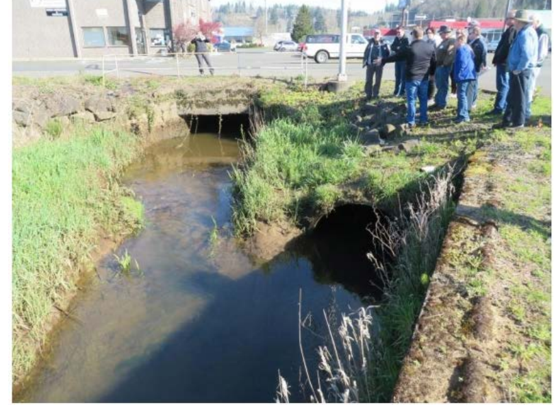
FRY CREEK - CULVERT CONSTRICTIONS
