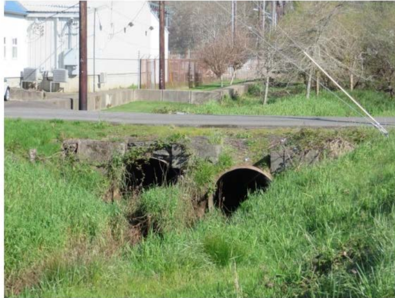
FRY CREEK - CULVERT CONSTRICTIONS
