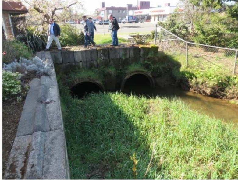
FRY CREEK - CULVERT CONSTRICTIONS
