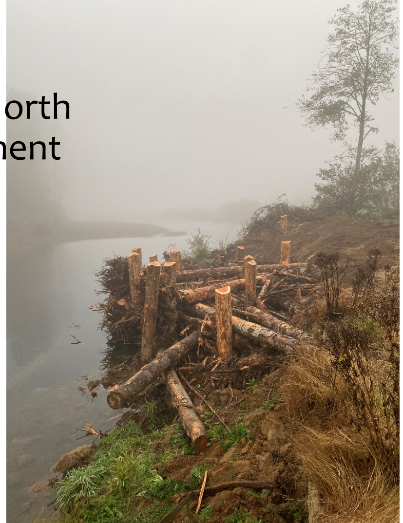
Deflector structures looking upstream
