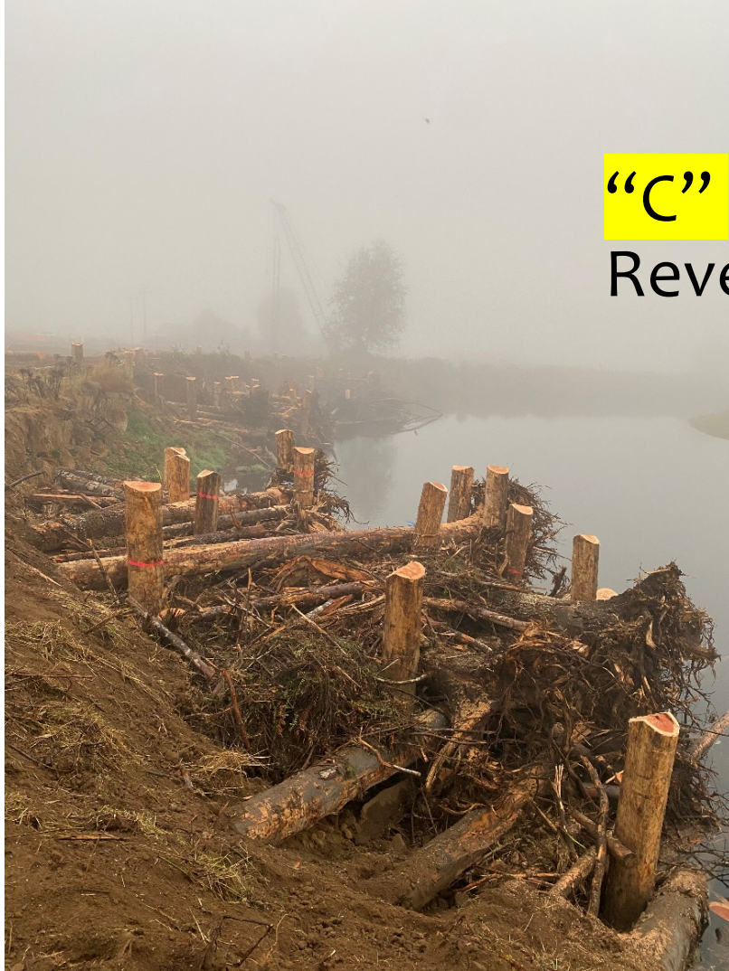
Deflector structures looking downstream
