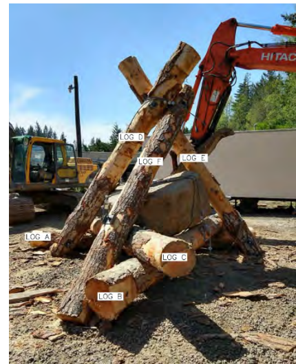
Figure 6 – Detail View of Log Jack, slash not shown
