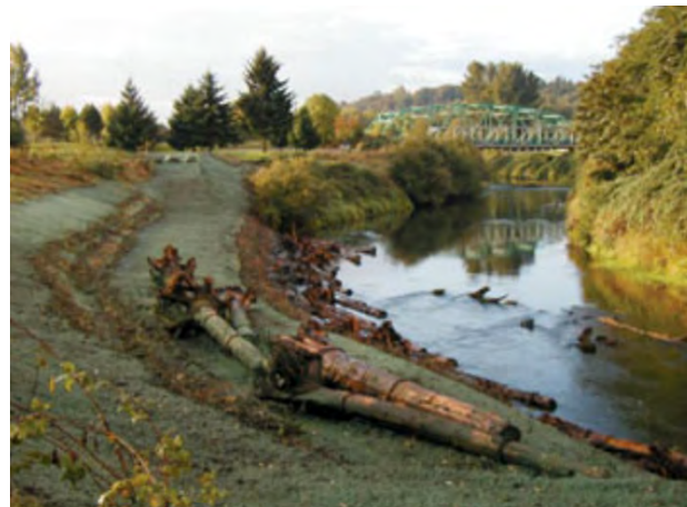
Figure 8 - Example of Log Rows (Photo: Green River Flood Control District)
