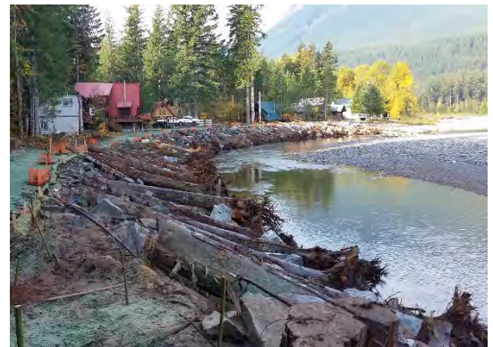
Figure 10 – Example of log revetment, Cowlitz River
