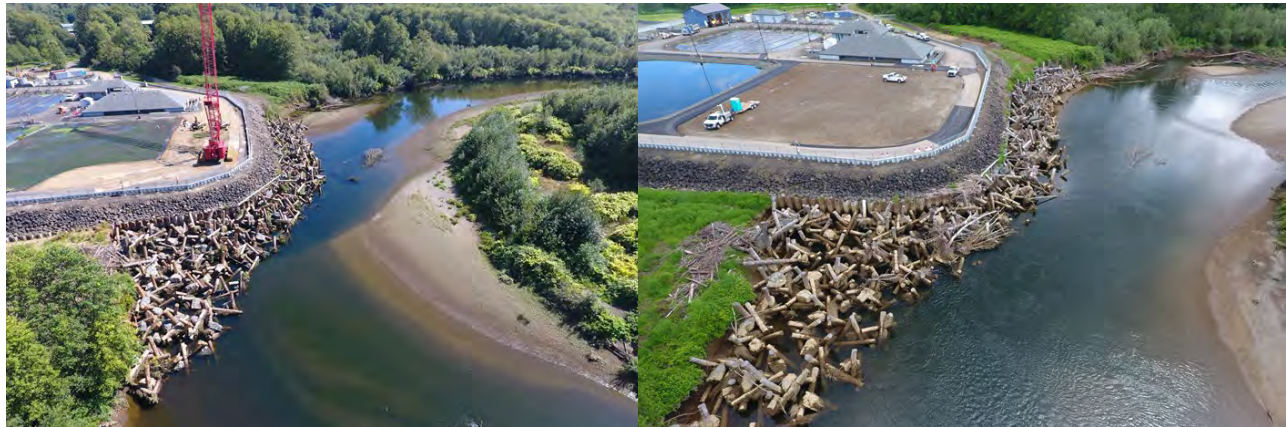
Figure 7 – Log Jacks immediately following installation on the Wynoochee River at Montesano WWTP (left) and one-year post installation (right.) Thalweg has shifted in the right photo.
