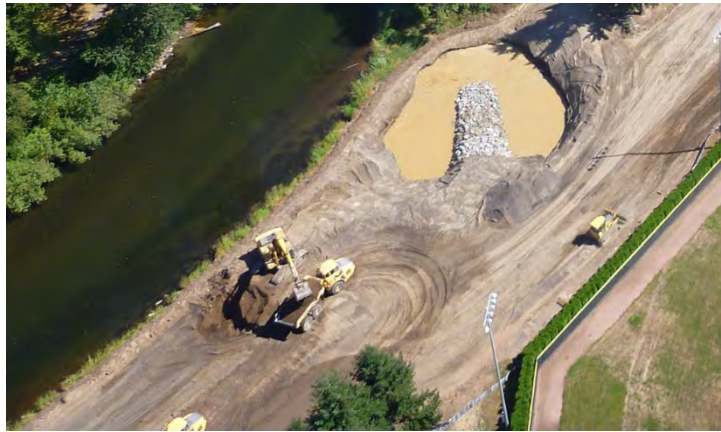
Figure 9 – Example of buried rock spur under construction, Green River.
