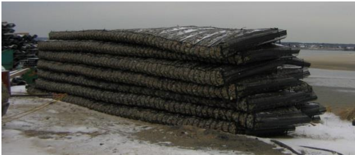
Figure 6 Stack of filled marine mattresses staged for placement on National Shoreline Erosion Control Development and Demonstration Program project in Seabrook, NH (photograph by Kevin Knuuti, CHL)
