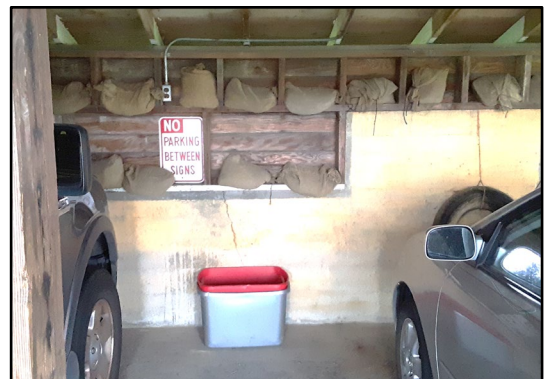
Mike stores filled sand bags on shelves and in nooks in his carport. Note the elevated electrical outlet above the sign.
