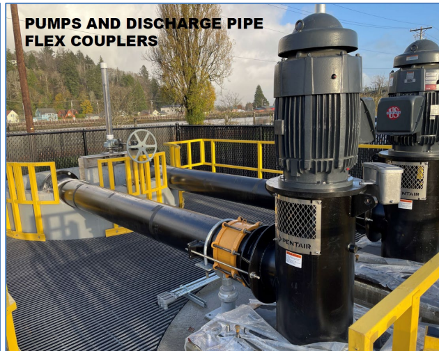
PROPELLER PUMP MOTORS INSTALLED
