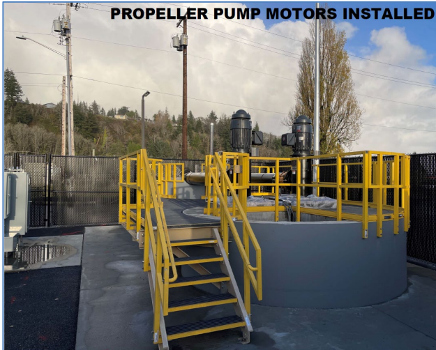
PROPELLER PUMP MOTORS INSTALLED
