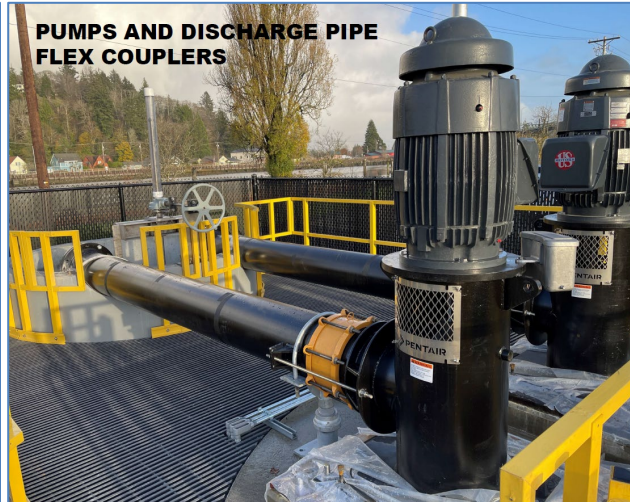
PROPELLER PUMP MOTORS INSTALLED
