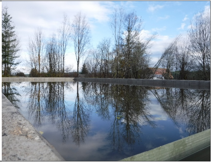
Boistfort Valley Water Pre-Sedimentation Pond, 2018 Photo Credit – Bob Amrine, Lewis County Conservation District
