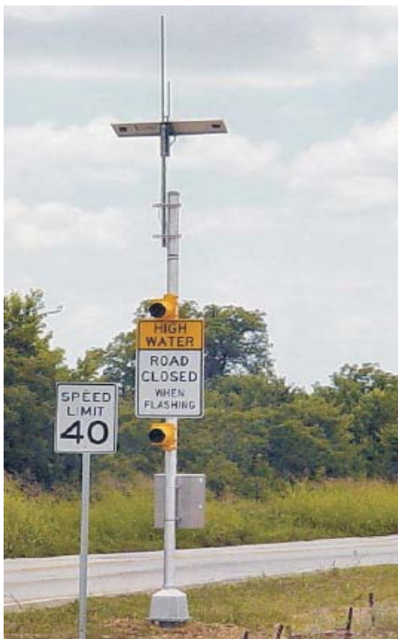
Figure - . Automated Road Closure Sign. (High Sierra Electronics Inc.)
