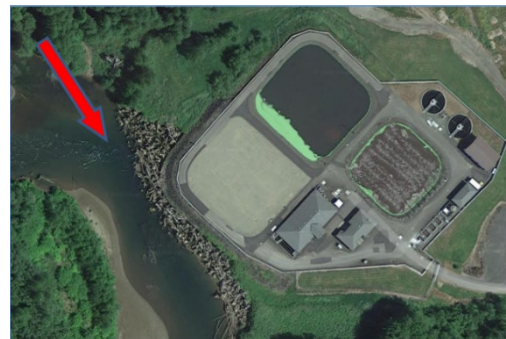
Figure 2 – After, October 2020 See Google Earth image here .
