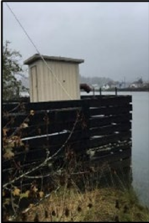
Pic 7 -- 10th St. Pump Station
