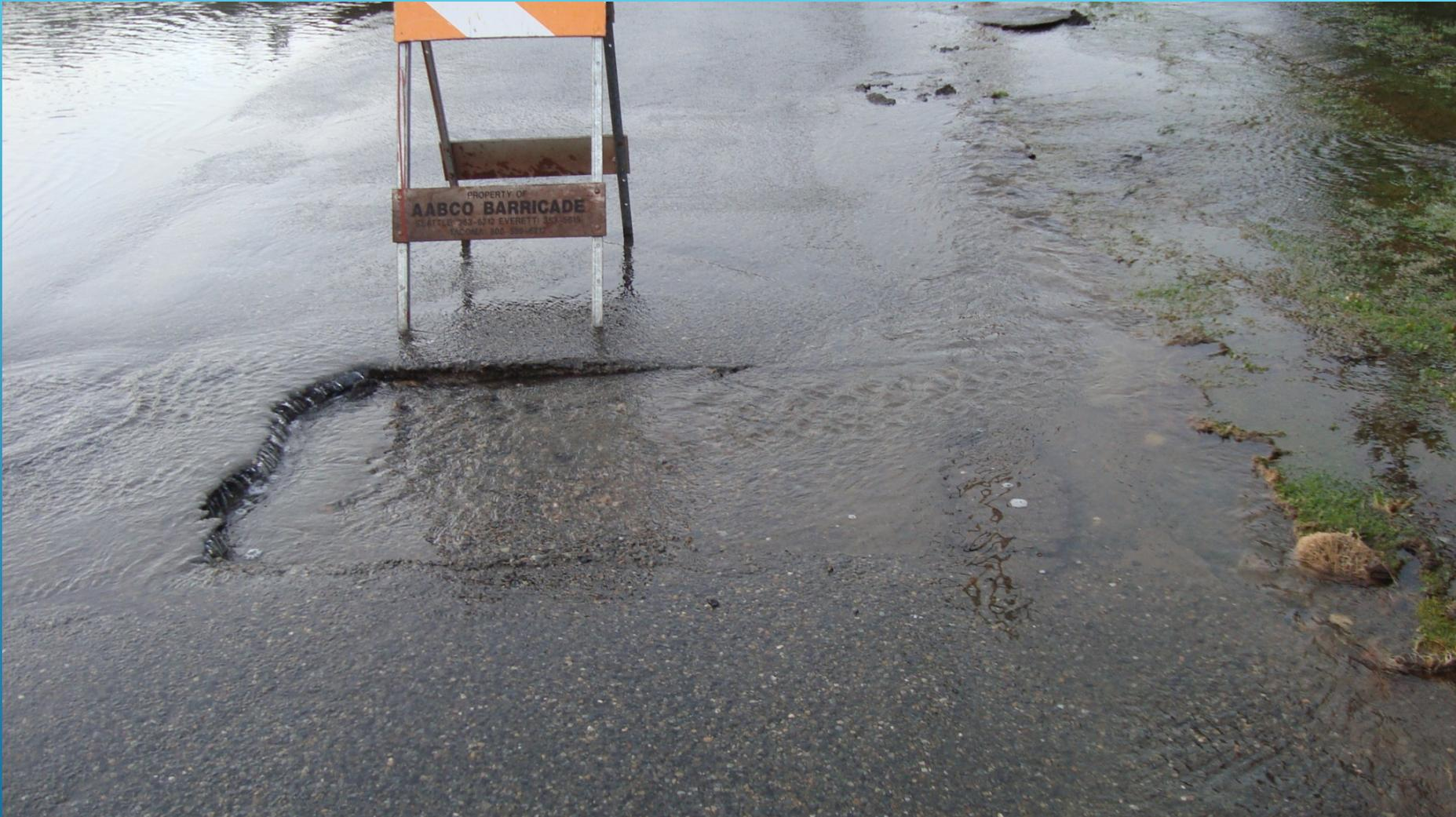
ASPHALT LIFTED AND DISPLACED NEAR 11<sup>TH</sup> AND MAIN STREETS
