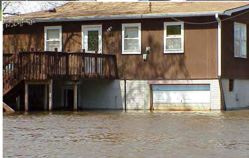
3.4. Protect for enclosures below the elevated floor
