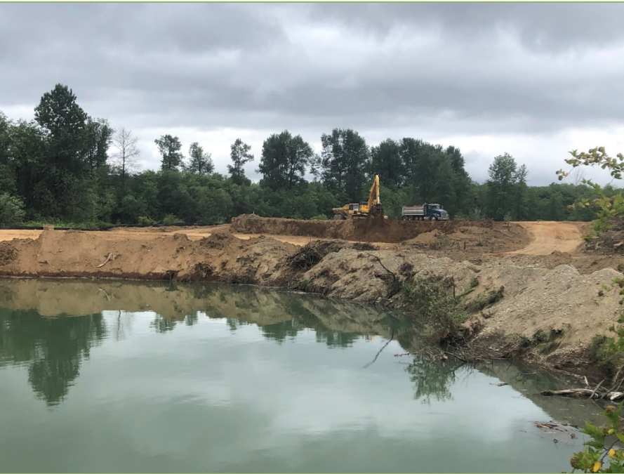
WDFW Ponds Restoration (remove spoils piles, shallow out ponds)
