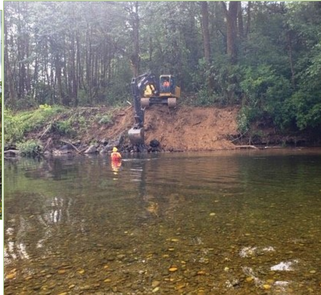
Lower WDFW Revetment (remove 200' rock toe, excavate 20' x 85' channel)
