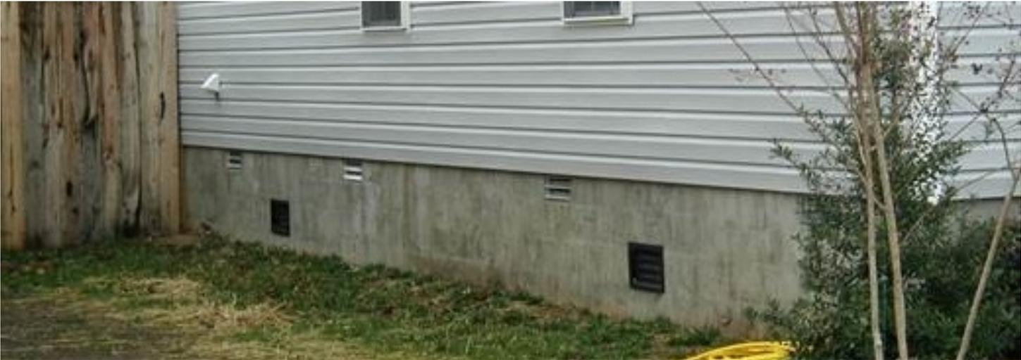
Example of Completed Retrofit (foundation has both air and flood vents)
