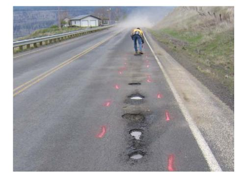
Many of QUADCO's roads that are not built to an All Weather Road Standard are either closed or restricted during the spring thaw. This can hinder the movement of goods and services. Improving the road's base and surfacing to an All Weather Road Standard solves this problem.
