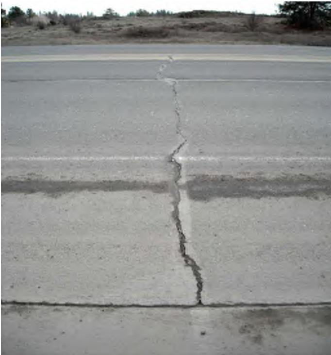
*Medium Severity Transverse Crack*
