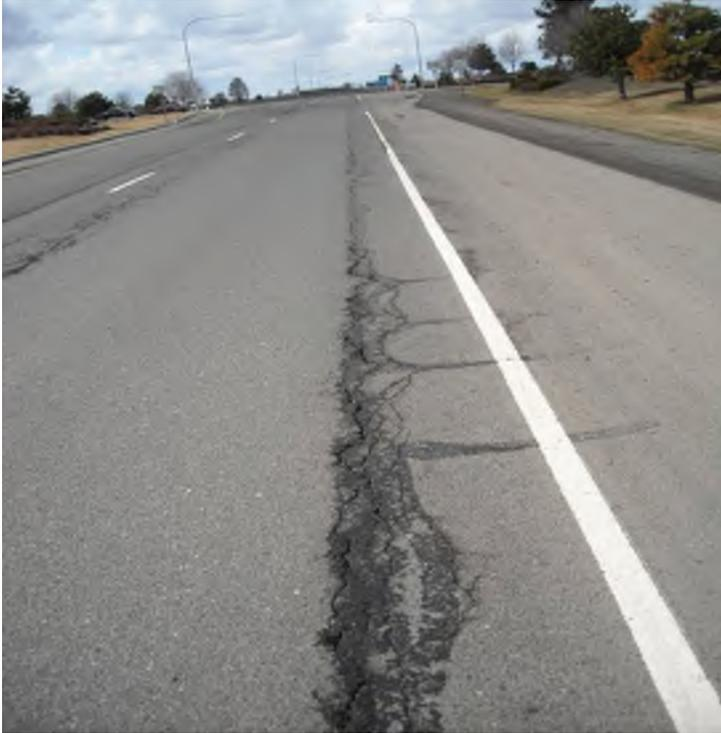
*High Severity Longitudinal Cracking*
