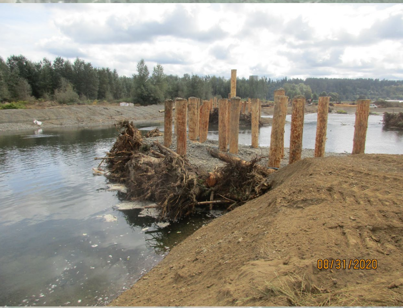
Lower Satsop Restoration and Protection Phase 1 2020-2021 Protection of Keys Road using log structures
