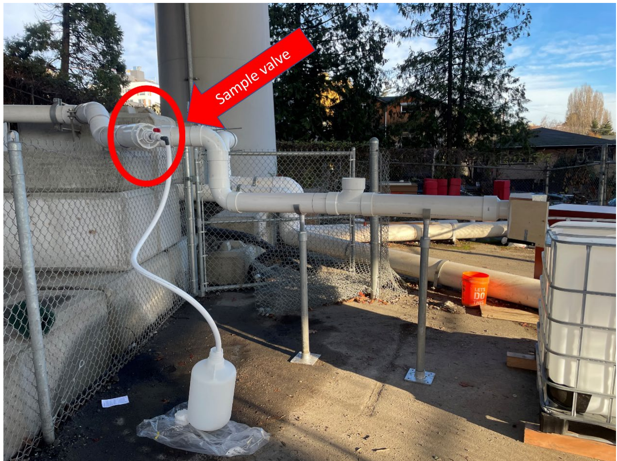
Figure 4. Sampling Valve and Illustration of Sample Collection
