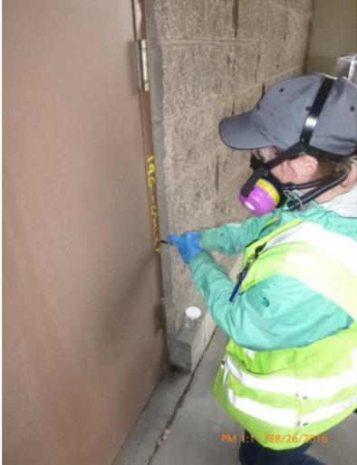
**The Boeing Company has removed over 23 miles of concrete joint compound at their Duwamish properties**
