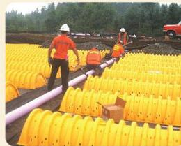
Installation of the infiltration chambers prior to re-seeding the grassy field.
