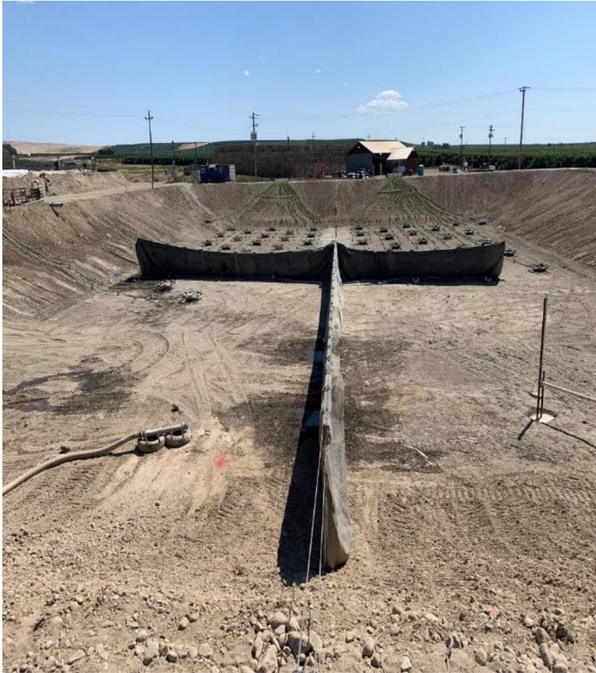
An existing dairy lagoon can be emptied and cleaned for insertion of floating baffles, micro-aerators, and recycle pumps to install a relatively low-cost NDN system on a dairy to **convert appropriately pre-treated liquid ammonia-N** to non-reactive nitrogen gas
