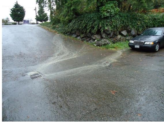
A turbid discharge was observed to a catch basin (see above photo). The source was identified as a failed temporary erosion and sediment control swale overflowing to the slope above the rockery (see photo below). The contractor employed Baker Tanks and pumps to eliminate the turbid flows.
