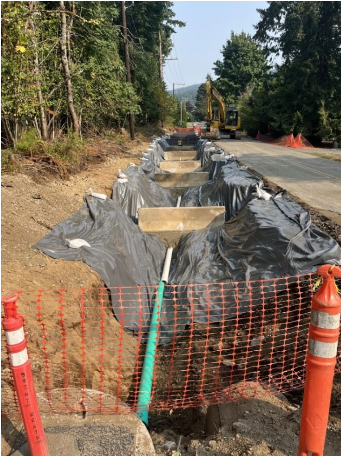
Figure B-1. Photograph of the “Austin South” Bioretention Swale Under Construction.
