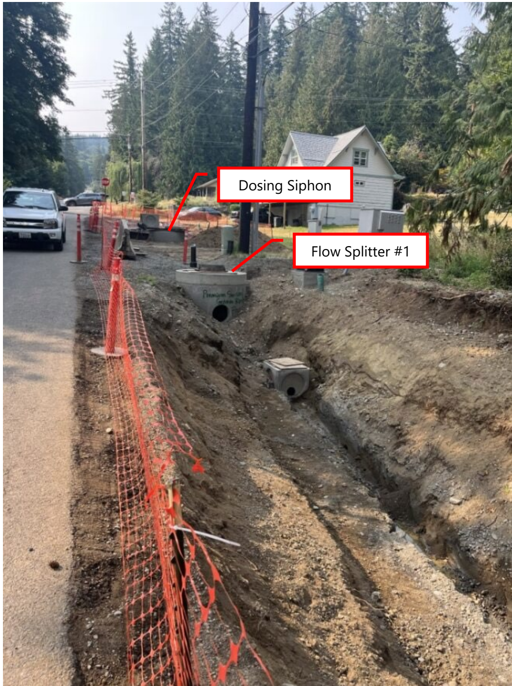
Figure B-2. Photograph of the "Austin South" Bioretention Swale Dosing Siphon and Flow Splitter #1.
